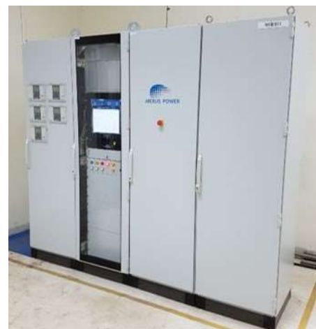
Fig. 2: New SVC control & protection system
