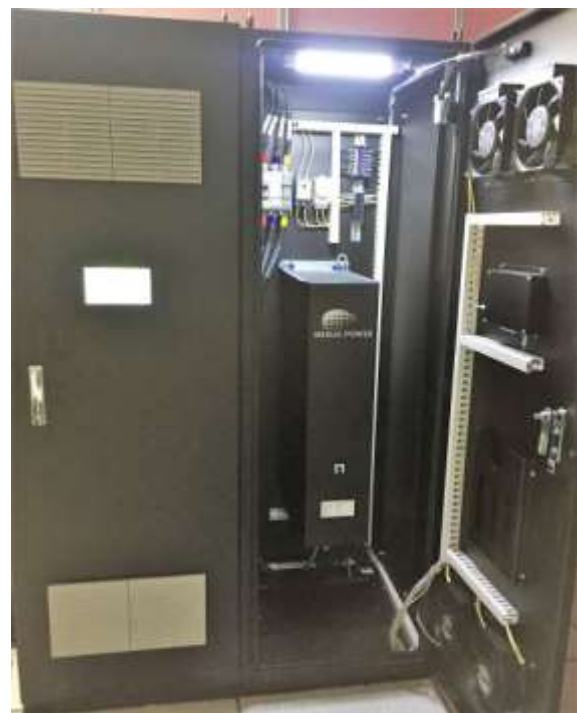
Fig. 3: AHF 380V 60Hz 100A located at 2AHF-2A panel
